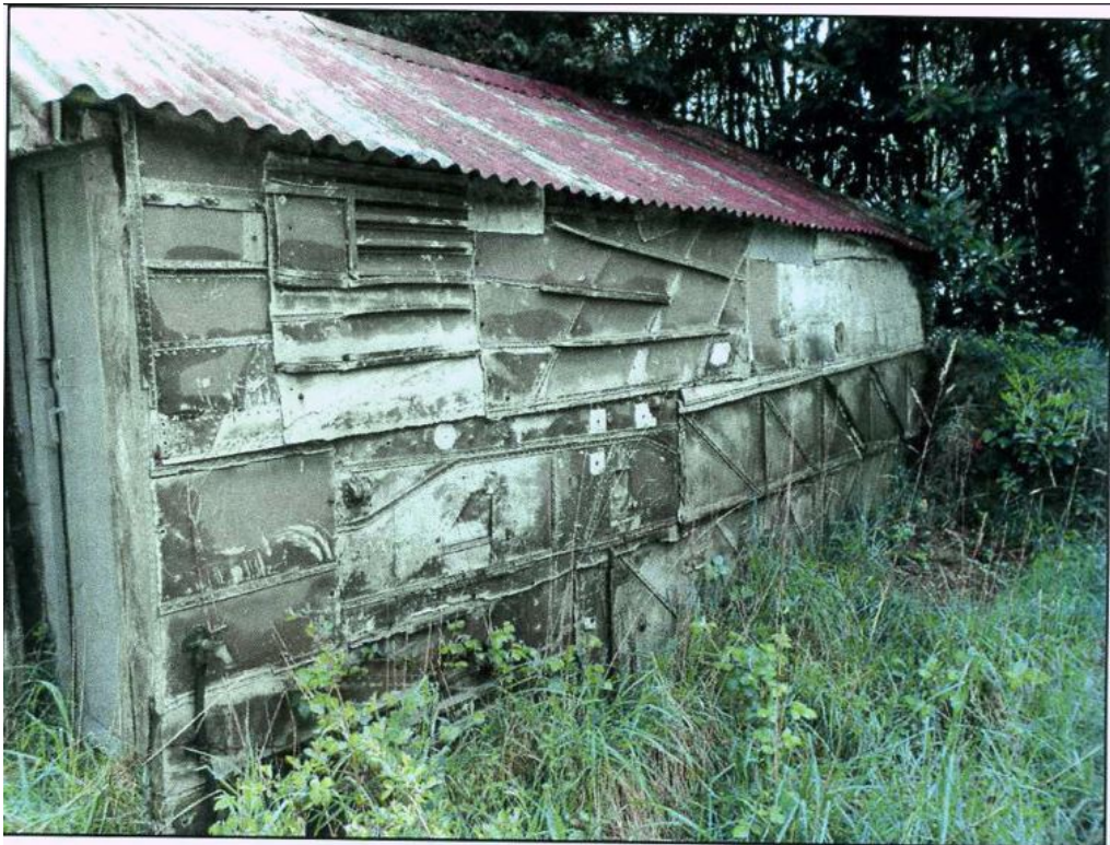
One of the sheds at Glomel with one wall made up entirely of Catalina components, at least some of which are from the internal wing structure Charles Street
